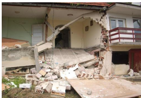
Fig. 7: Material damage in slope zones of Tuzla
