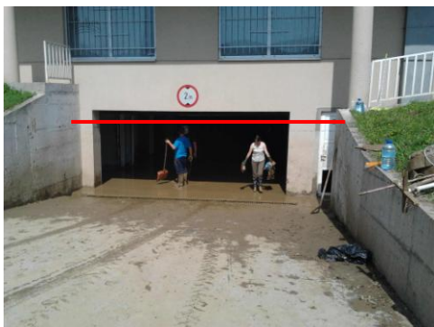
Fig. 5: Tuzla, Irac settlement, august 2014. (water level in basement rooms – red line)
