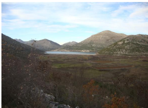
Fig. 2. End of Popovo field valley in Hutovo with visible remains of former abyss. Now karst cracks are injected with concrete basin, which present Trebišnjica's water reservoir, as well as reservoir for reversible water from Svitavsko lake created from HPP "Čapljina"
